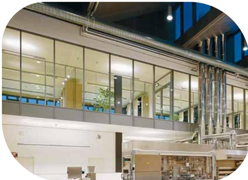
Pilkington **Pyrostop**® consists of multiple laminates of float glass and a special transparent intumescent interlayer, which is totally compatible and optically homogeneous with the glass. When exposed to fire, the pane facing the flames fractures but remains in place. As the heat penetrates the glass, the interlayers, one after the other, react by foaming to form a thick, opaque, resilient and tough insulating shield that blocks the conductive and radiant heat of the blaze.
