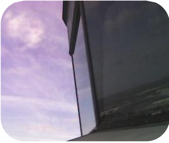
Exterior view showing glass tilted out at the top of an aircraft control tower.
