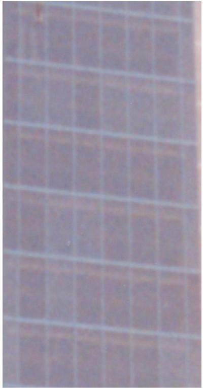
Example of 10 mm (3/8") thick, single glazed tempered glass, with irregular orientation. About 20 lights are perceptibly darker. This condition created a customer complaint. (The unenhanced photograph of an eastern elevation, was taken in grey sky conditions near dawn)
