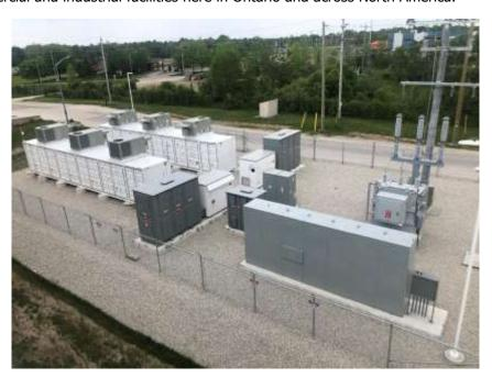
Above: The batteries reduce how much power the Collingwood plant pulls from the grid whenever peak times are predicted.
