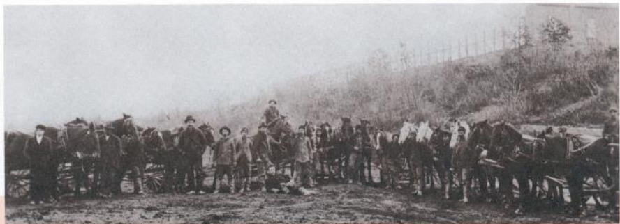
Breaking ground for Edward Ford's new plant at Rossford
