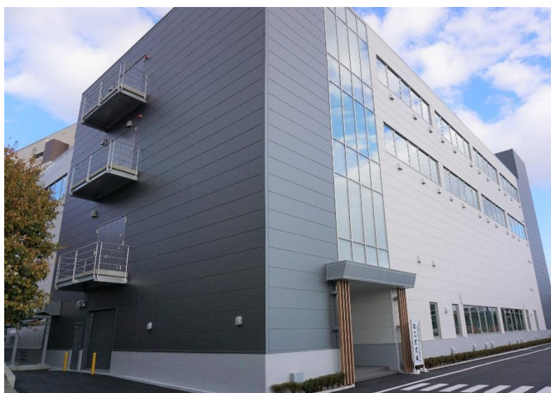
Second Research Building
