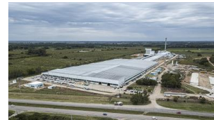
New float furnace in Argentina
