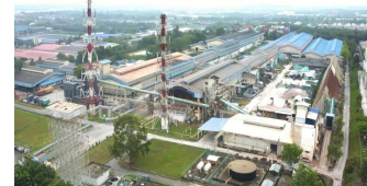
Float furnace in Malaysia
