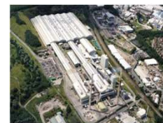
Greengate site (UK) where rolled glass and float glass capacities being integrated
