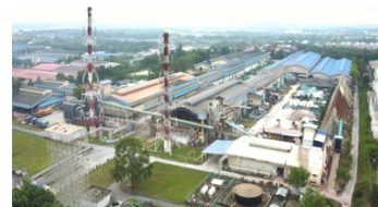
Float furnace in Malaysia
