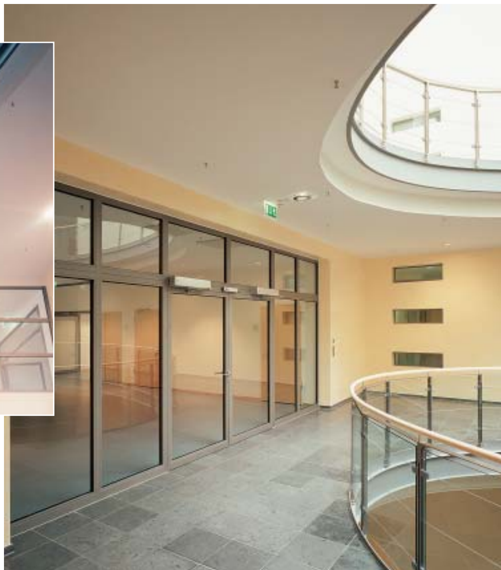
Extensive transparent fire lobbies opening onto the atrium are constructed on each floor with F 30/T 30/RS door systems.
