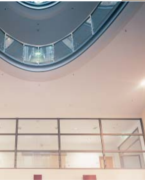
View of the foyer in the inner core of the building with its central atrium: the transparent walls of the escape routes and emergency walkways are built from Pilkington Pyrostop™ glass to fire resistance class F 30 (Jansen system).
