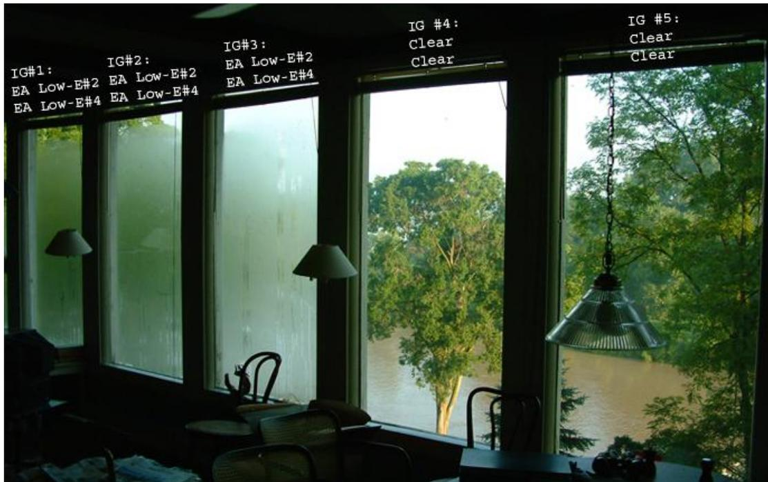
First surface condensation on three high performance North elevation, river facing, windows. Ohio, 7:30 a.m. in June. Still air, 70 °F inside and outside, 85% Relative Humidity, 65 °F Dew Point.
