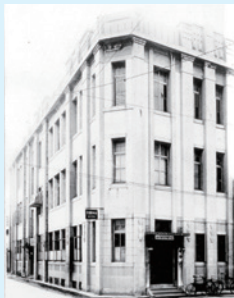
the office building at the time of foundation (which later became the head office)
