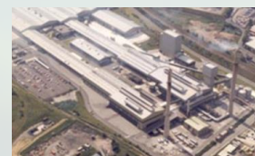
Greengate site, St. Helens, UK
