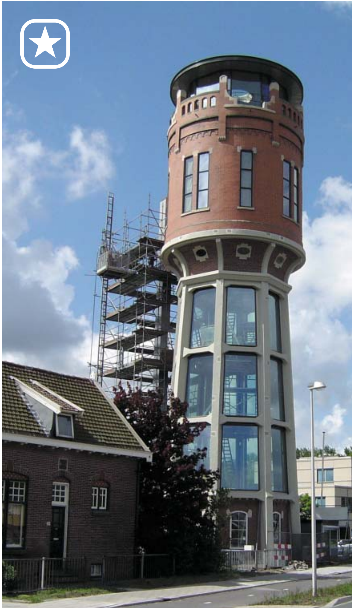
Water Tower, Hazerswoude-Rijndijk , Netherlands
